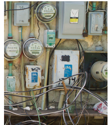
Right: A tangle of wires creates an on-site hazard.
